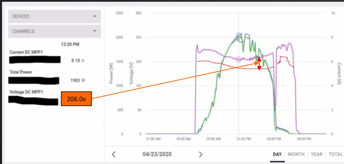
Performance: MPPT DC Voltages drop
